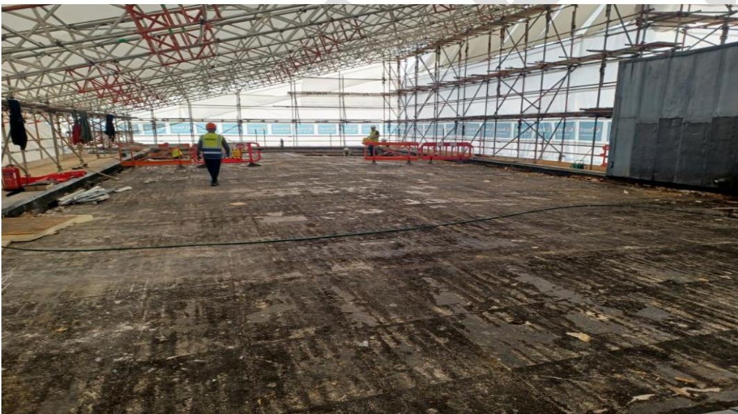
Images above: progress on Town Centre House
